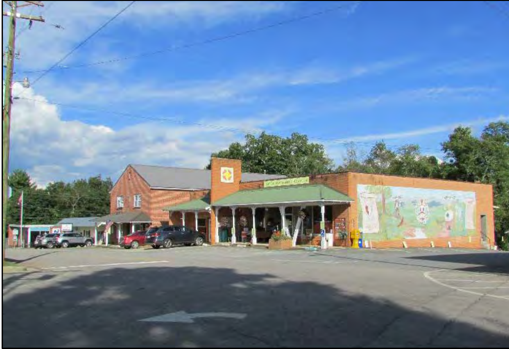
Figure 66. 96 and 104 Sanderson Street, now the Clay County Chamber of Commerce and Masonic Lodge No. 301.
