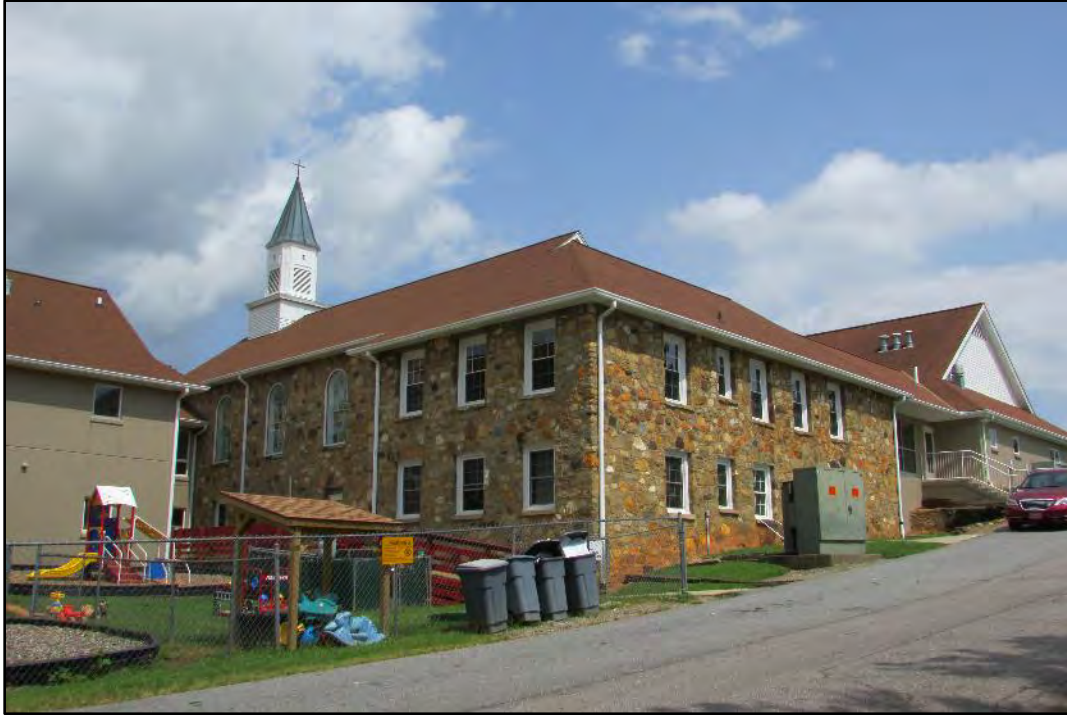
Figure 25. Hayesville United Methodist Church, looking east toward original portion of northwest and southwest (rear) elevations.
