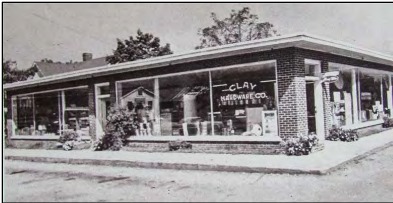
Figure 48. Clay Hardware Company, 61 Main Street, date unknown (Courtesy of Historic Hayesville, Inc.).
