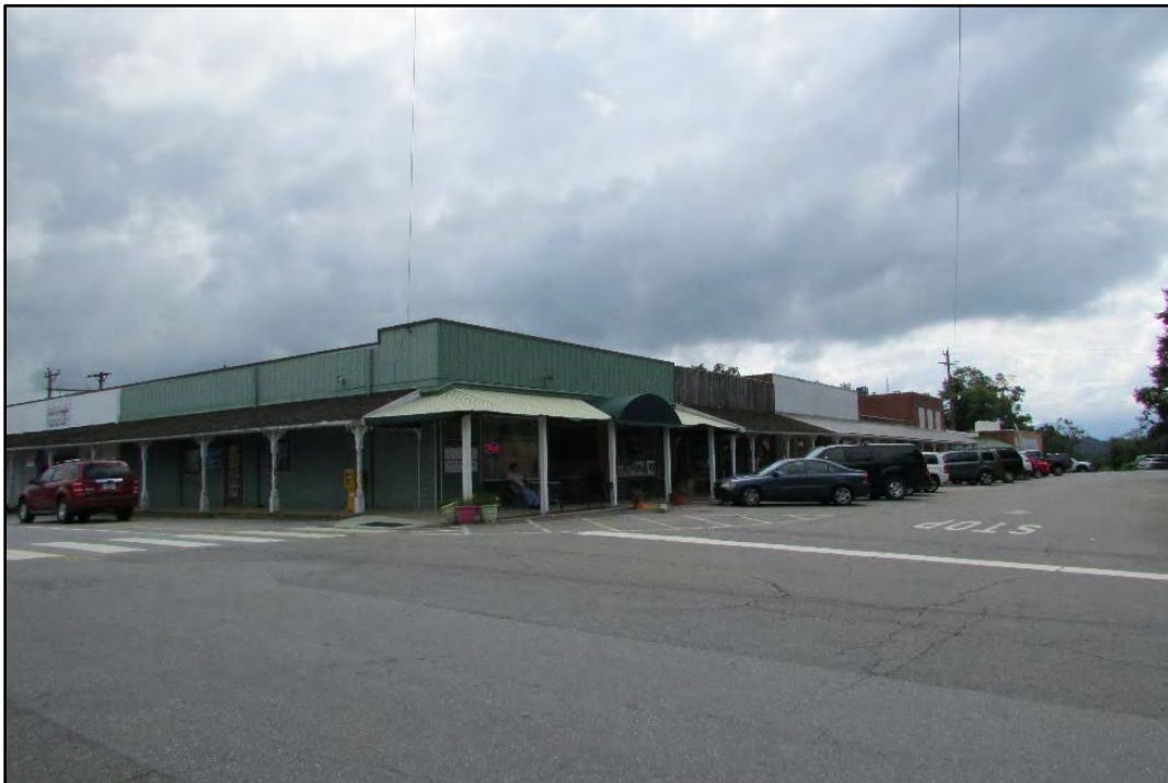
Figure 70. North side of Church Street between Sanderson and Main Streets, looking northeast.
