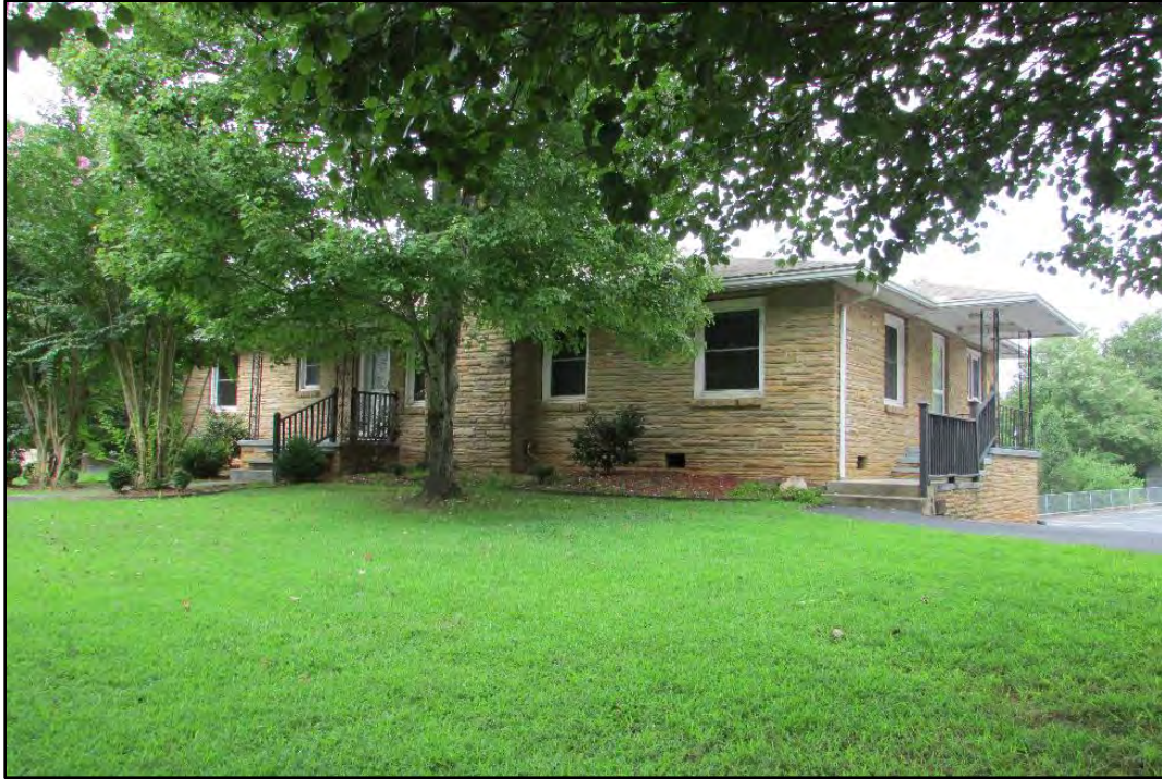
Figure 15. Truett Memorial Baptist Church parsonage, south and east elevations, looking northwest.
