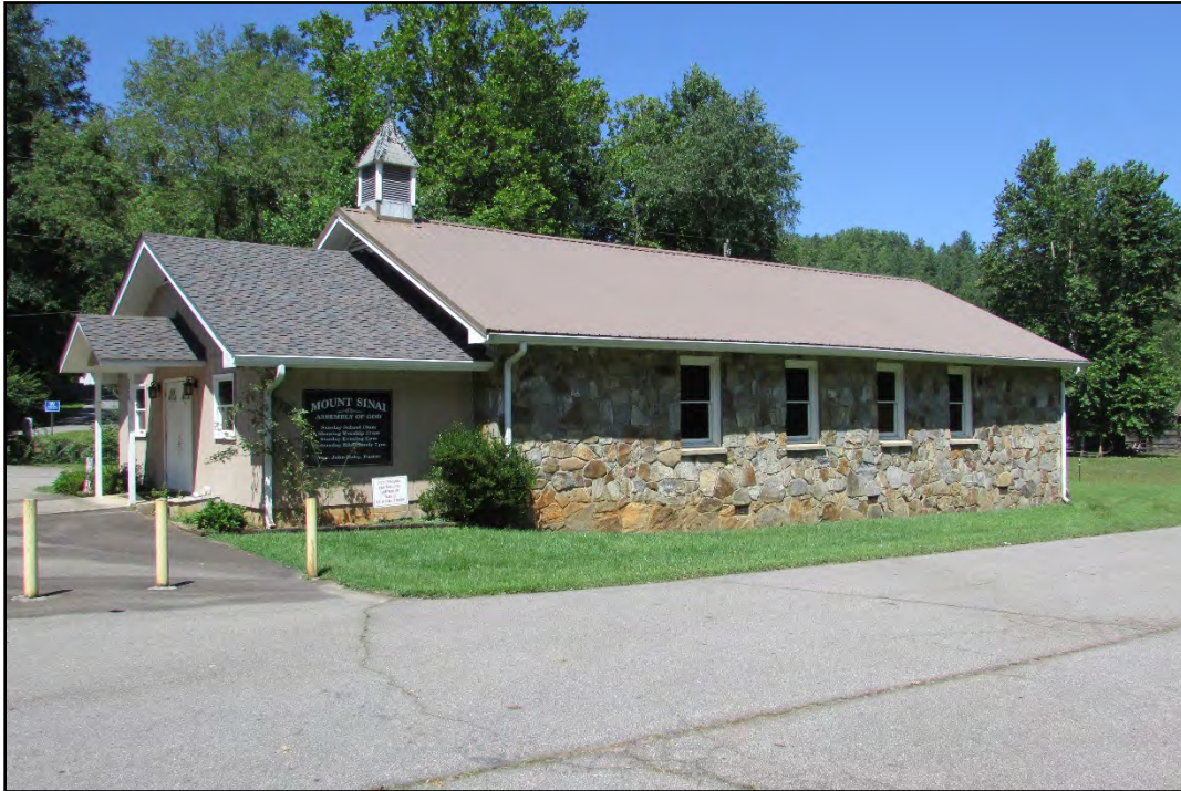
Figure 36. Mount Sinai Church (MA334), 5869 Upper Burningtown Road, Franklin, Macon County, looking northeast.
