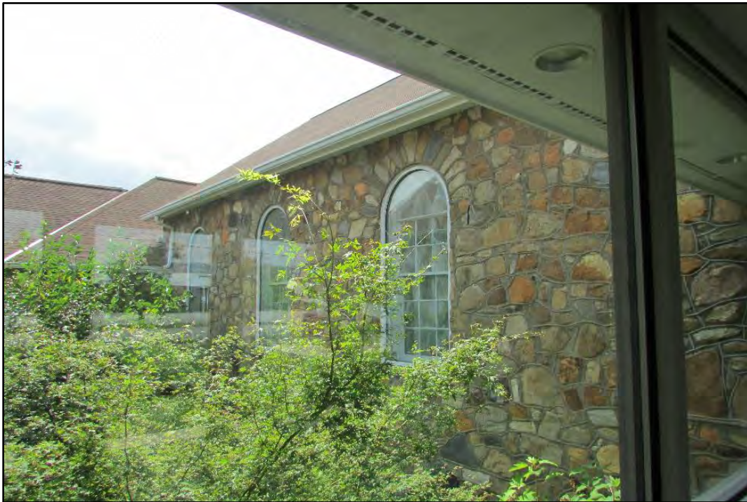
Figure 30. Hayesville United Methodist Church, looking southwest from inside the 2004 sanctuary connector wing toward the southwest elevation of original sanctuary.
