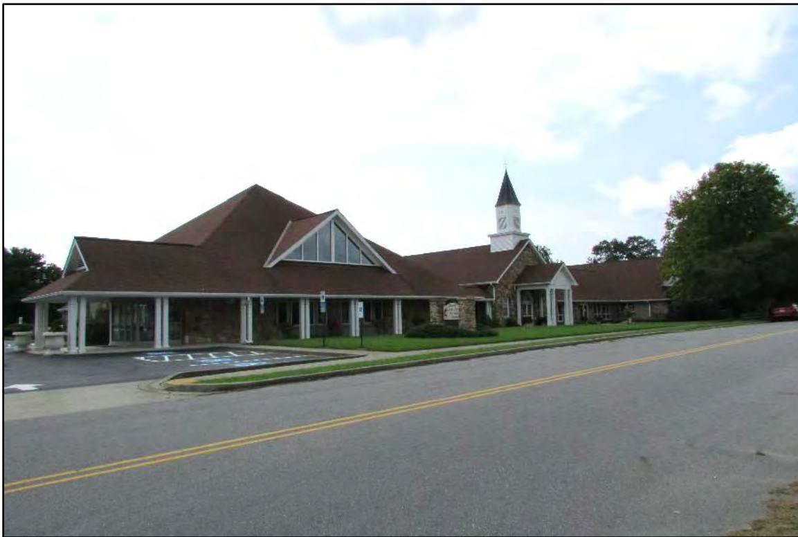
Figure 21. Hayesville United Methodist Church (CY0061), front (northeast) elevation.
