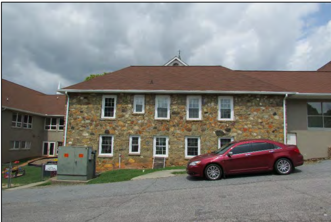
Figure 26. Hayesville United Methodist Church, looking northwest toward original portion of southwest (rear) elevation.
