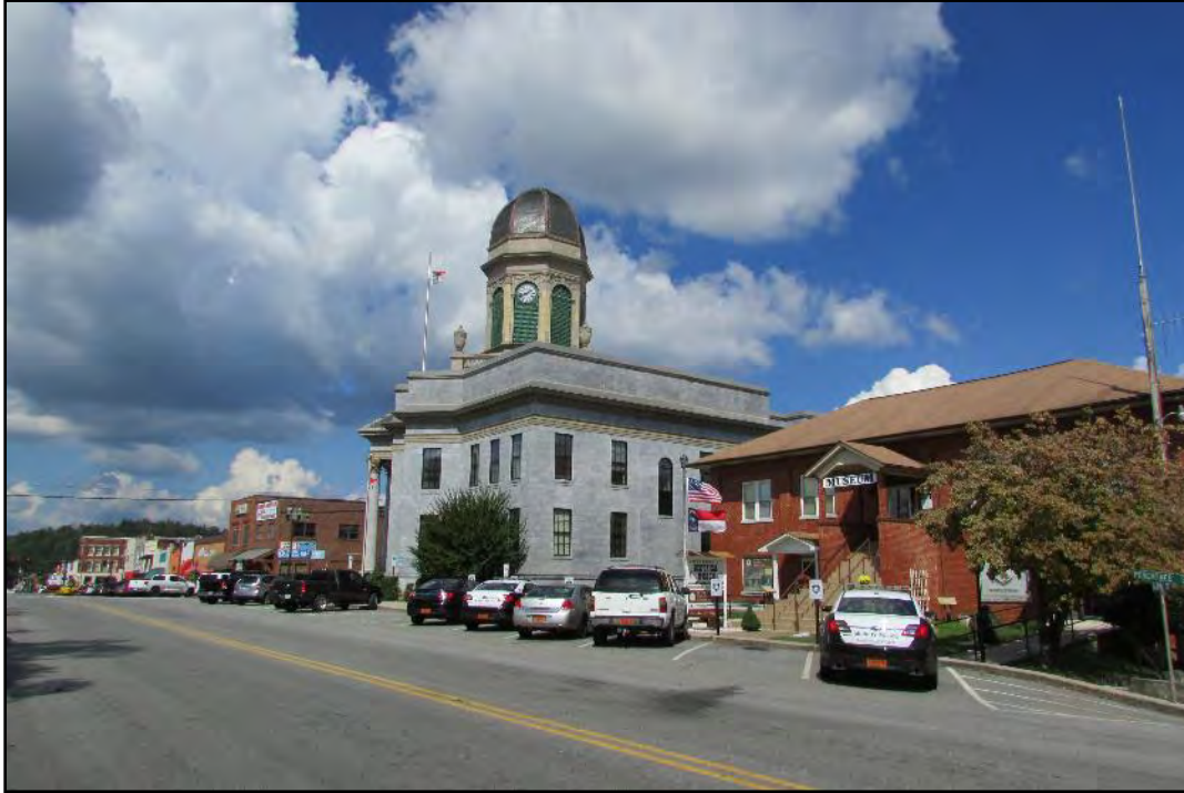
Figure 72. Downtown Murphy and the Cherokee County Courthouse, Peachtree Street from Alpine Street, looking northwest.
