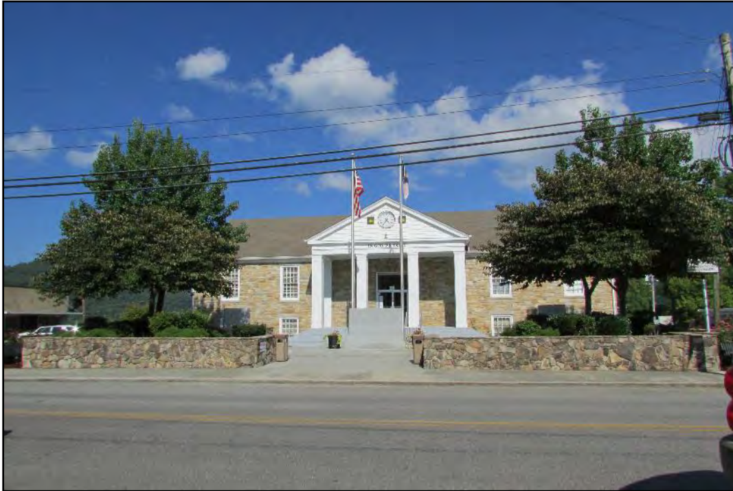
Figure 73. Graham County Courthouse, North Main Street, Robbinsville, looking east.
