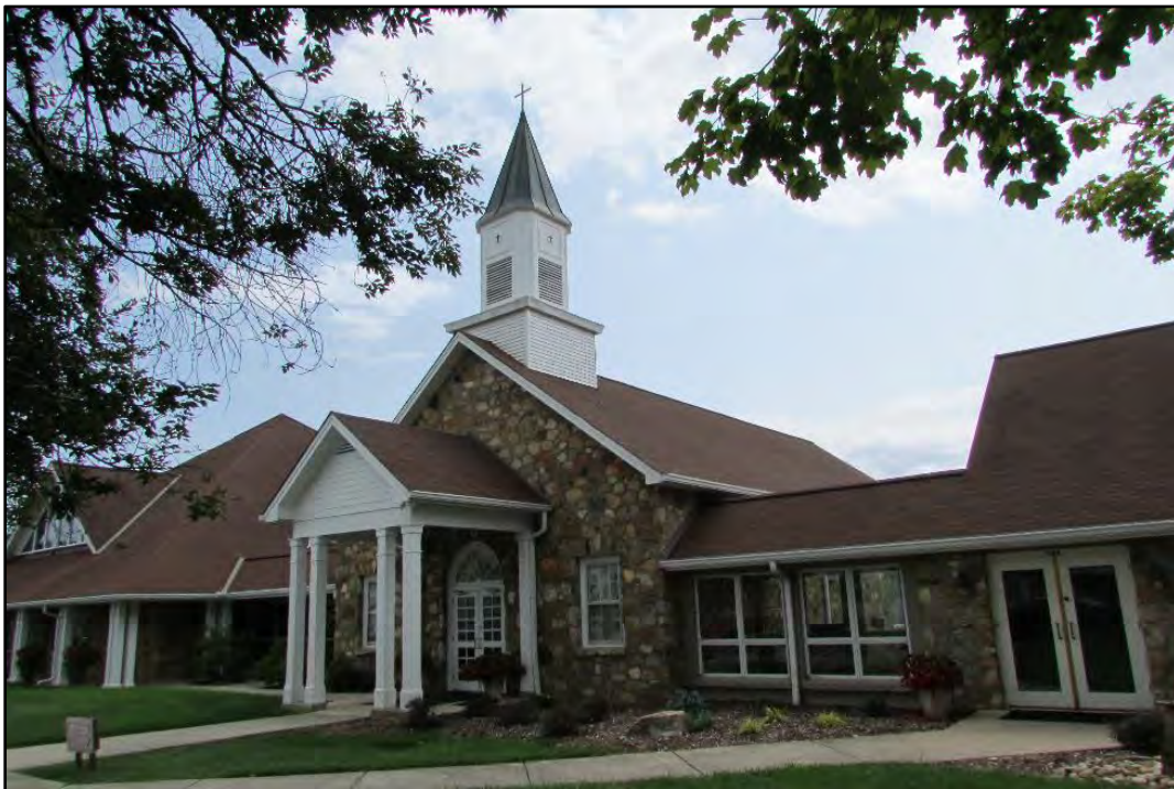
Figure 29. Hayesville United Methodist Church, looking southeast toward original sanctuary and connecting hyphen to new sanctuary.
