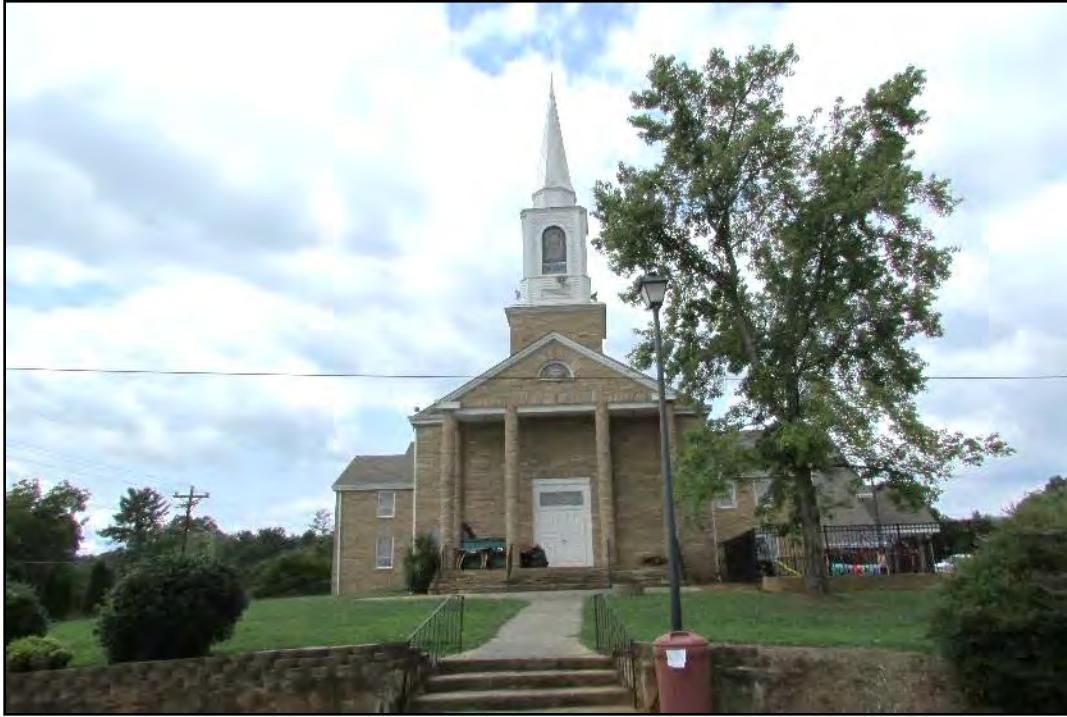
Figure 5. Truett Memorial Baptist Church, front (southeast), looking northwest.
