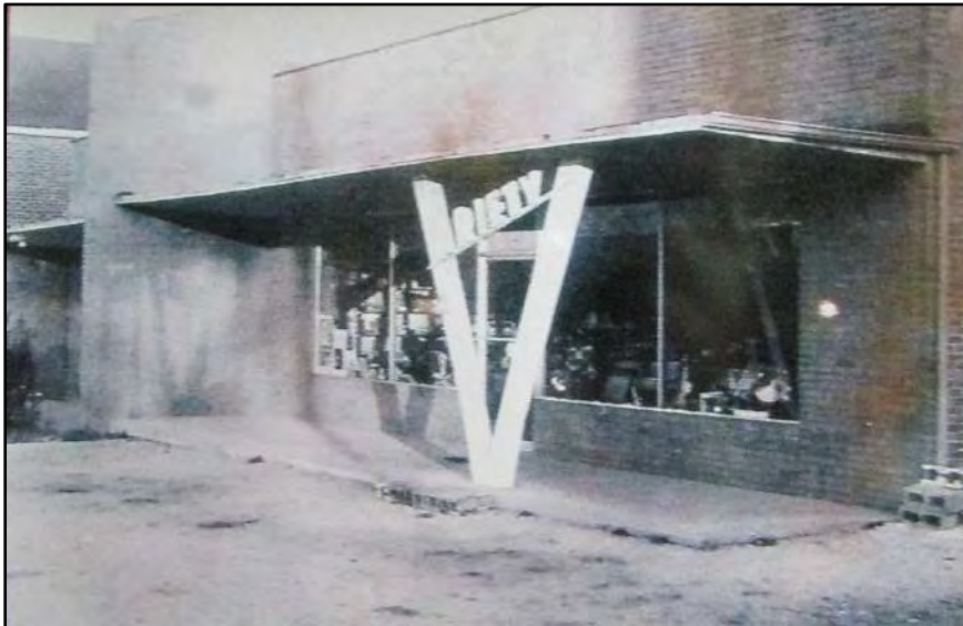
Figure 65. Eva's Variety Store, 96 Sanderson Street, date unknown (Courtesy of Historic Hayesville, Inc.).
