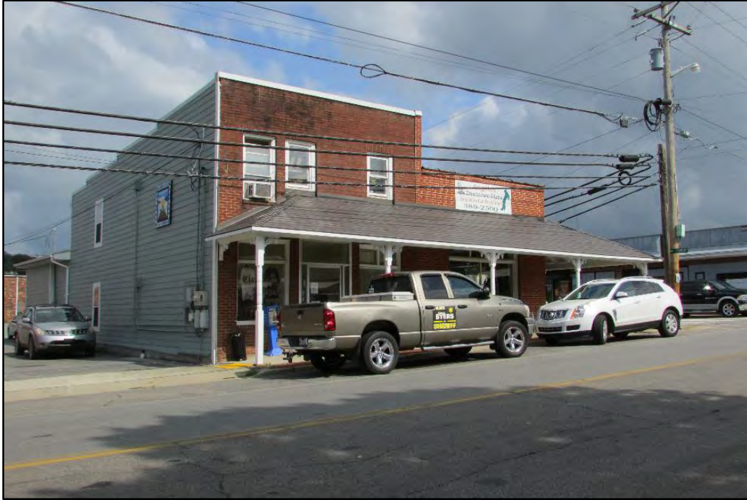
Figure 51. 43-45 Main Street, looking northwest. Now occupied by Angelo's and Clay County Progress.
