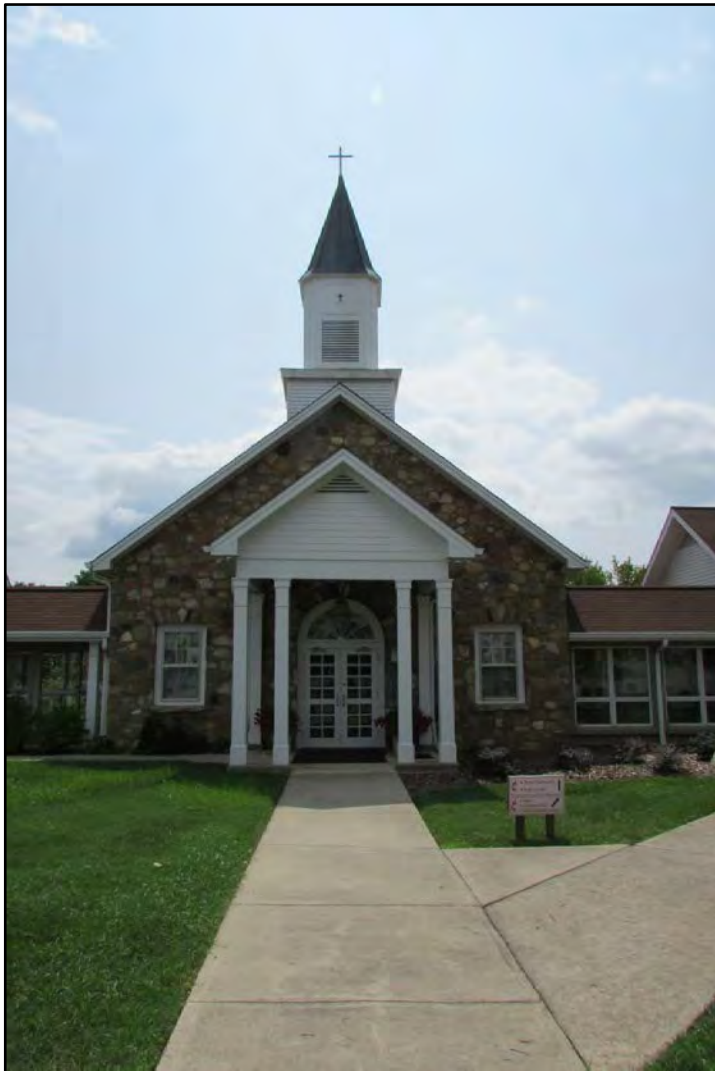
Figure 24. Hayesville United Methodist Church, looking southwest toward the façade of original sanctuary.
