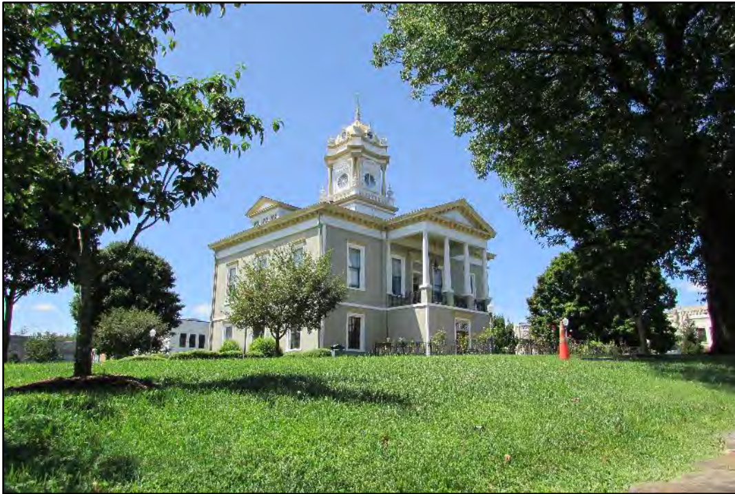
Figure 75. Burke County Courthouse, Morganton, South Green Street, looking west.
